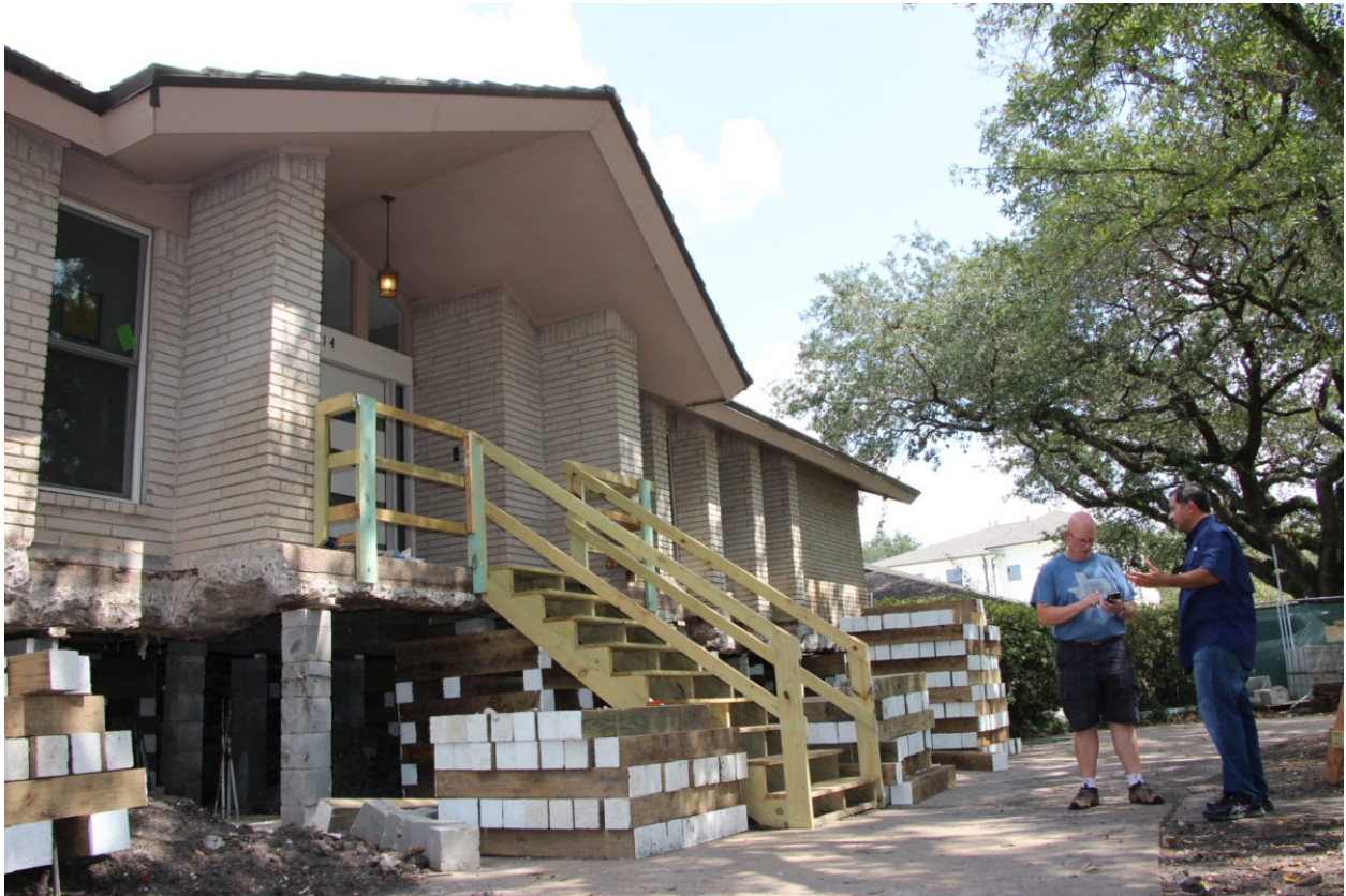
Figure 1: Floodproofing in Houston, TX ( Houston Public Media )
